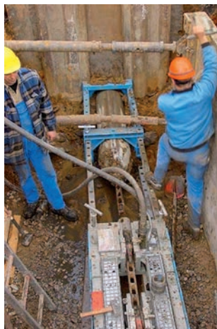
Pitless pipe laying with vonRoll ECOPUR pipes.
